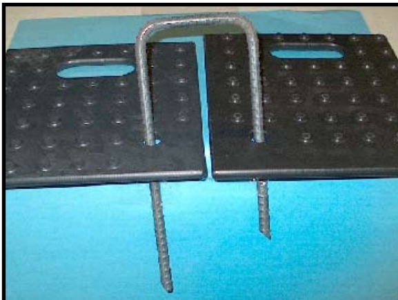
Step 3: Place stake through holes and pound into soil using Sledge Hammer.
